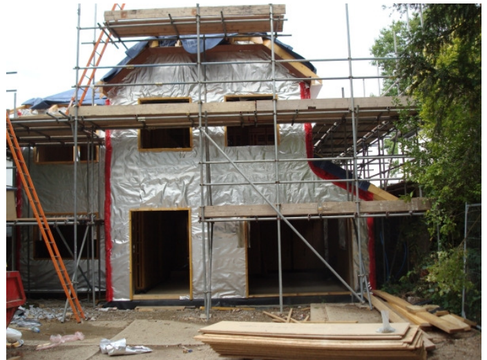
The erected and breather-papered SIP Frame
